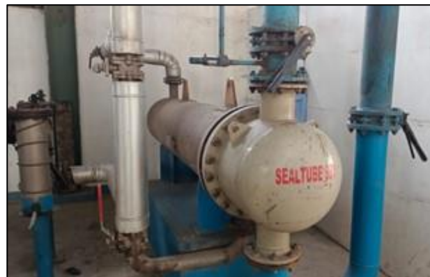
Gambar 1. Heat Exchanger Sealtube 881X
