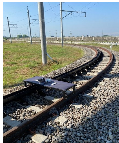
Figure 1. Design of unmanned rail inspection.
