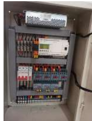
Figure 3. Installation of electrical components and wiring
