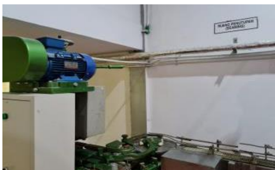
Figure 2 Signs on every process rooms
