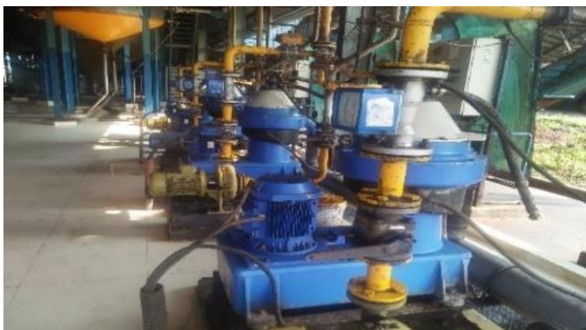
Gambar 1 Mesin purifier (PAPX 317 SGD 11-G)
